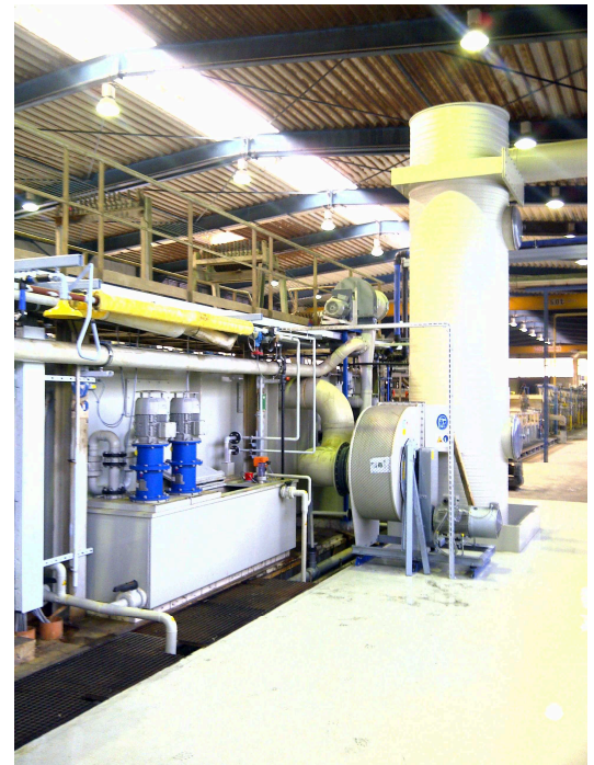
EXHAUST AIR SCRUBBER WITH FAN
